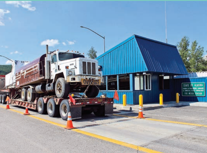
Fox Weigh Station; photo by Matthew Matta, ADOT&PF.
