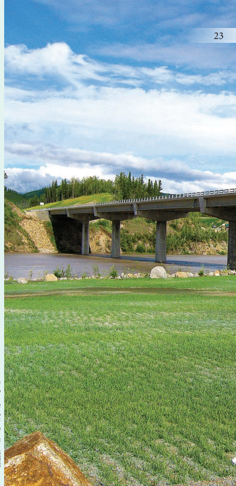
New Tanana River Bridge, Elmer Marx, ADO18PF
