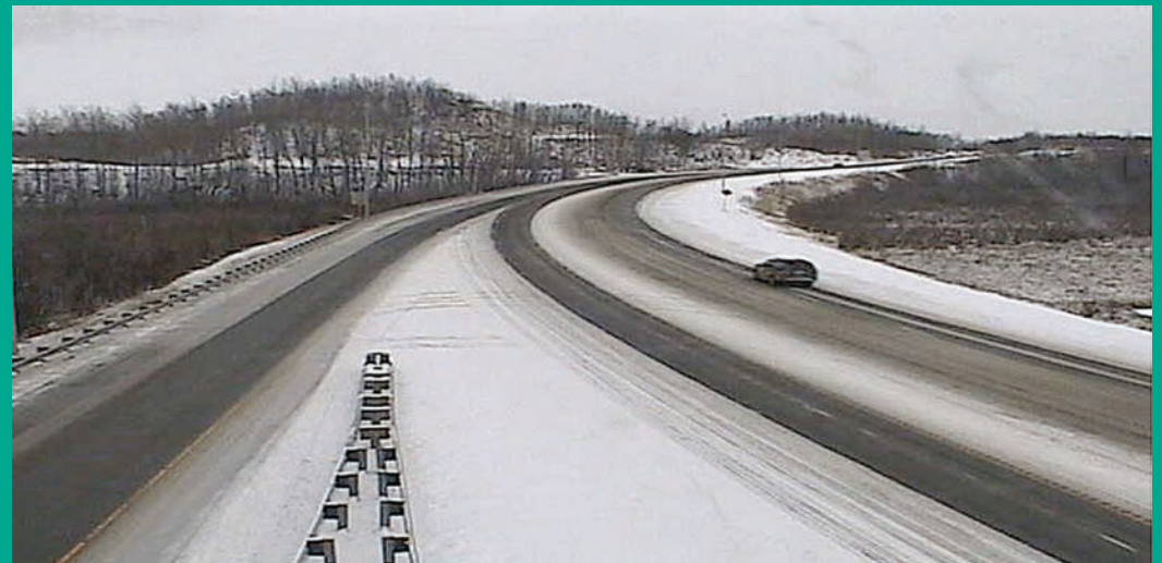
511 Road Information camera image, MP 35.8 Glenn Highway, ADOT&PF.
