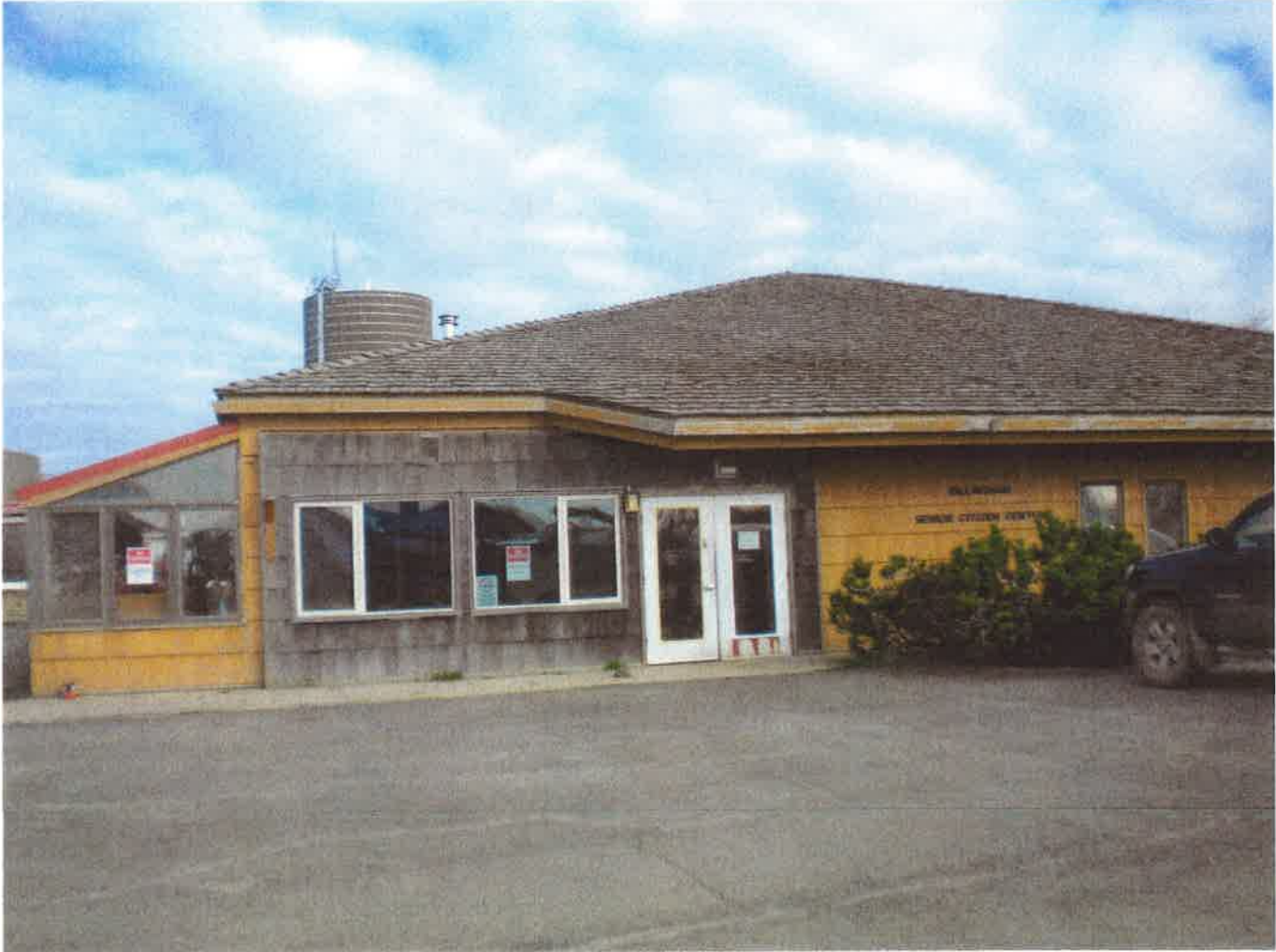
Dillingham Senior Center front entrance. Areas for safely loading and off-loading passengers for single vehicles, the Dillingham Senior Service vehicles and the Aleknagik Senior Services vehicles is provided.
