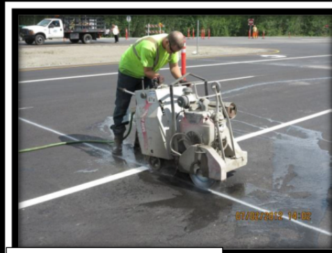
Saw cutting post construction
