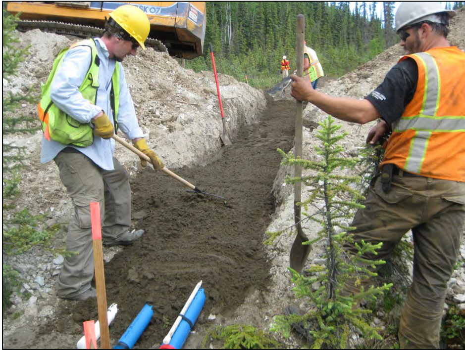
Figure C-3. Covering the casings with sand bedding. (Photograph by M. Darrow, June 2012)
