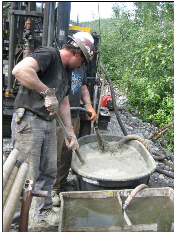
Figure B-6. Preparing the cement-bentonite grout for backfill into TH10-1553. (Photograph by M. Darrow, June 2010)
