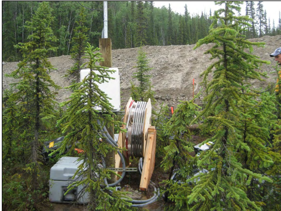
Figure C-11. Installation of SAA device, showing shipping reel position relative to embankment and ADAS. (Photograph by M. Darrow, July 2012)
