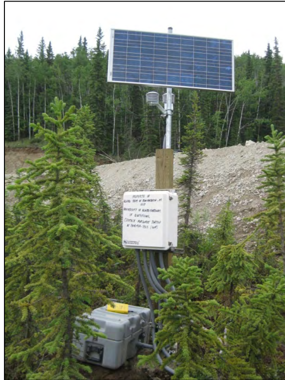
Figure C-26. Final ADAS configuration located near the downslope toe of the embankment. The thermal berm is visible behind the ADAS. (Photograph by M. Darrow, July 2012)
