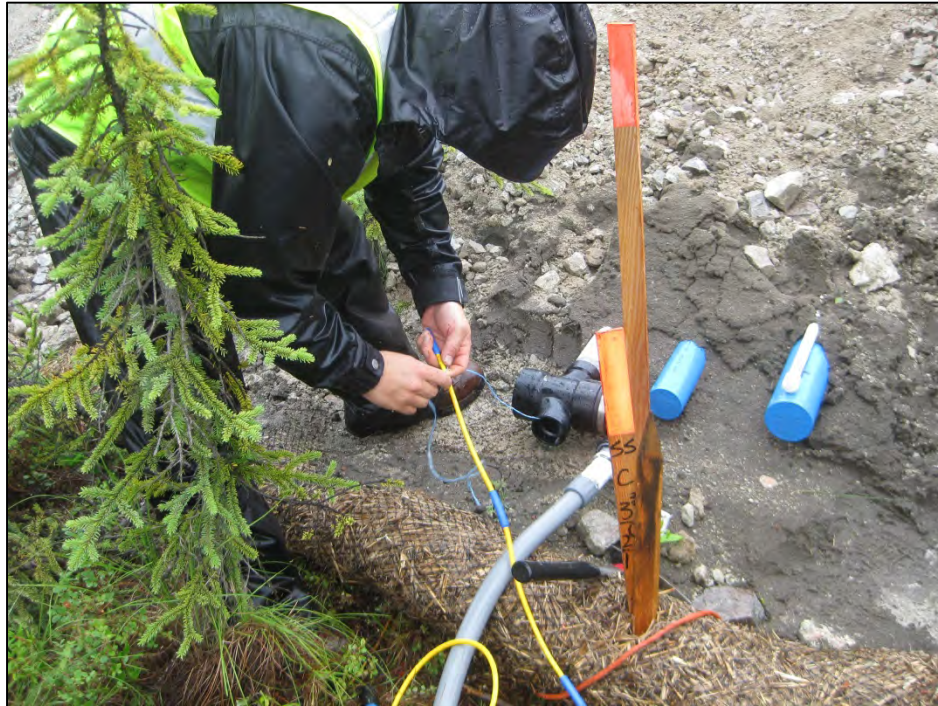
Figure C-7. Attaching the pull rope to the end of the TAC device. (Photograph by M. Darrow, July 2012)
