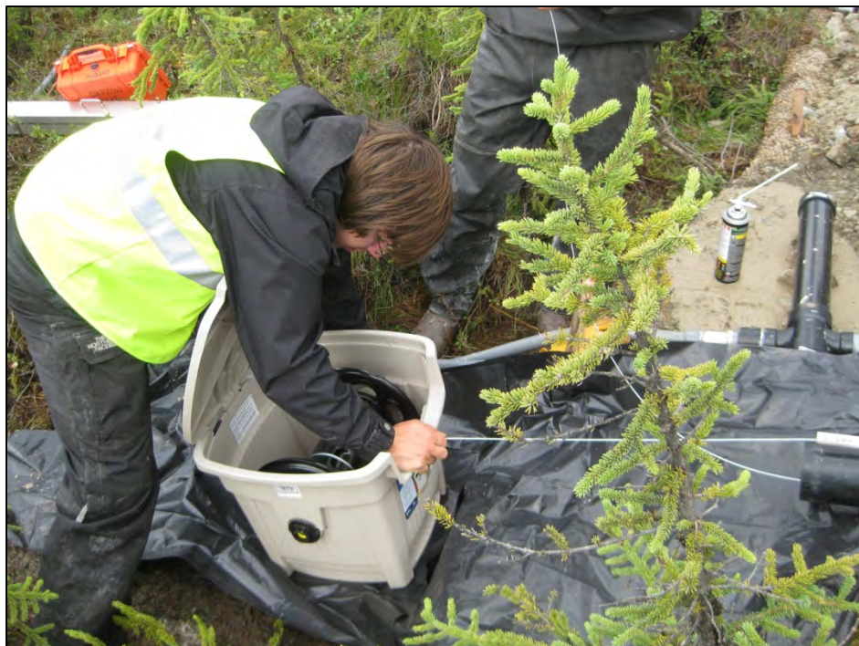
Figure C-21. Winding up excess wire rope from within casing assembly. (Photograph by M. Darrow, July 2012)
