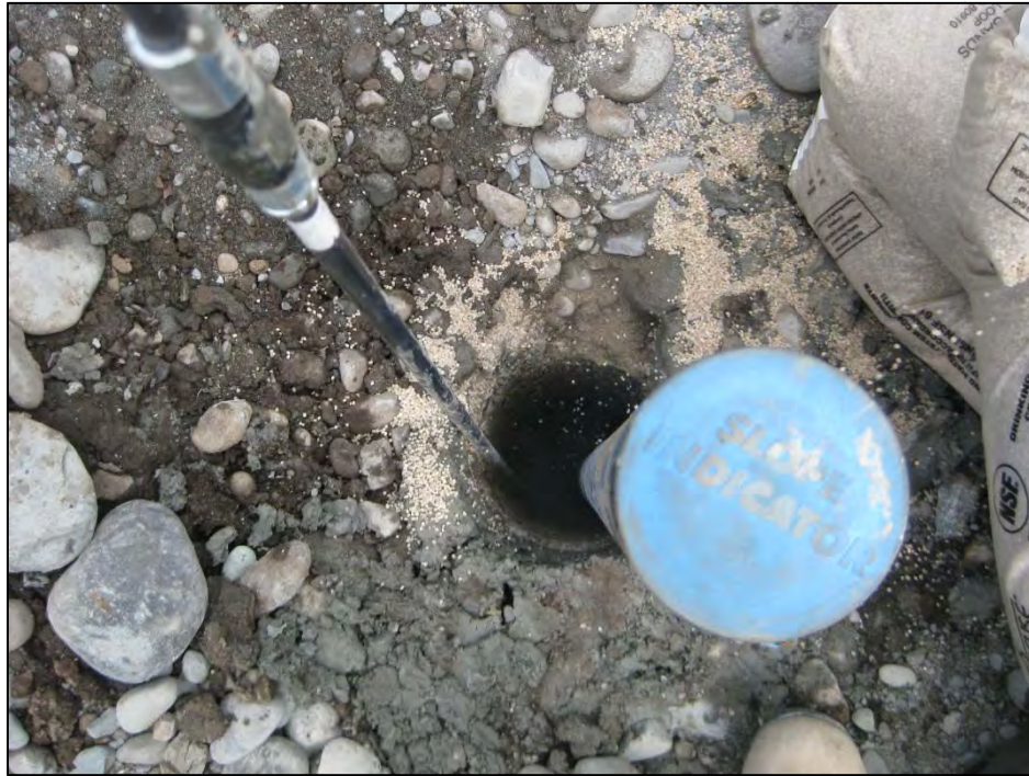
Figure B-1. Tamping dry sand backfill around the guide casing. (Photograph by M. Darrow, June 2010)
