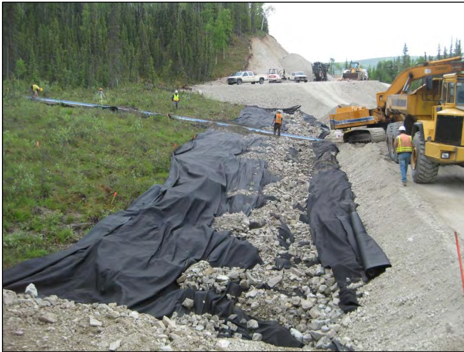
Figure C-1. Looking southeast towards the instrumented cross section. Geotextile with some ACE material is present in the foreground. (Photograph by M. Darrow, June 2012)
