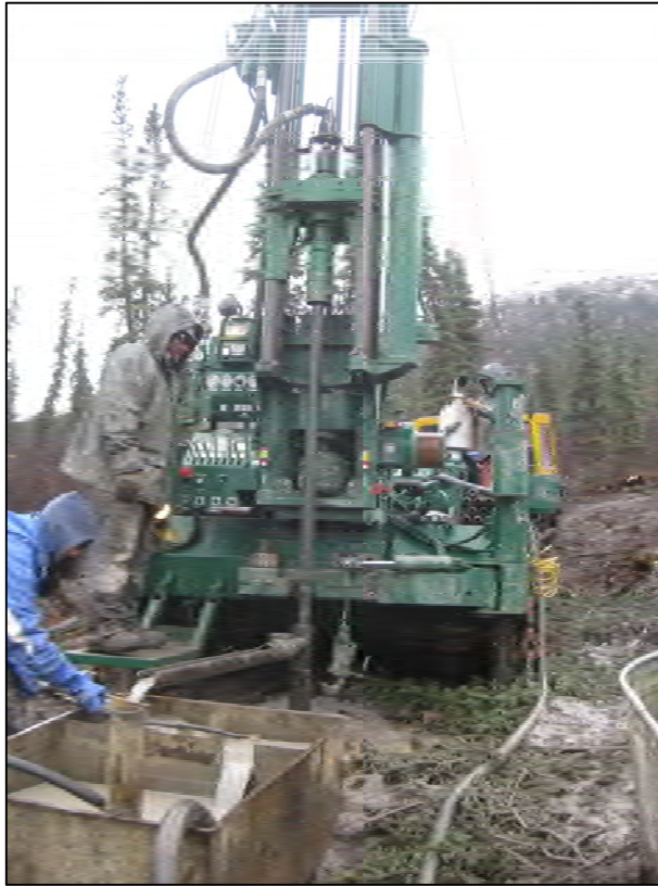
Figure D-1. Drilling TH12-9004 with tricone and casing. (Photograph by M. Darrow, Sept. 2012)
