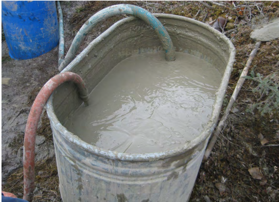
Figure D-2. Cement-bentonite grout during the back-filling process. (Photograph by M. Darrow, Sept 2012)
