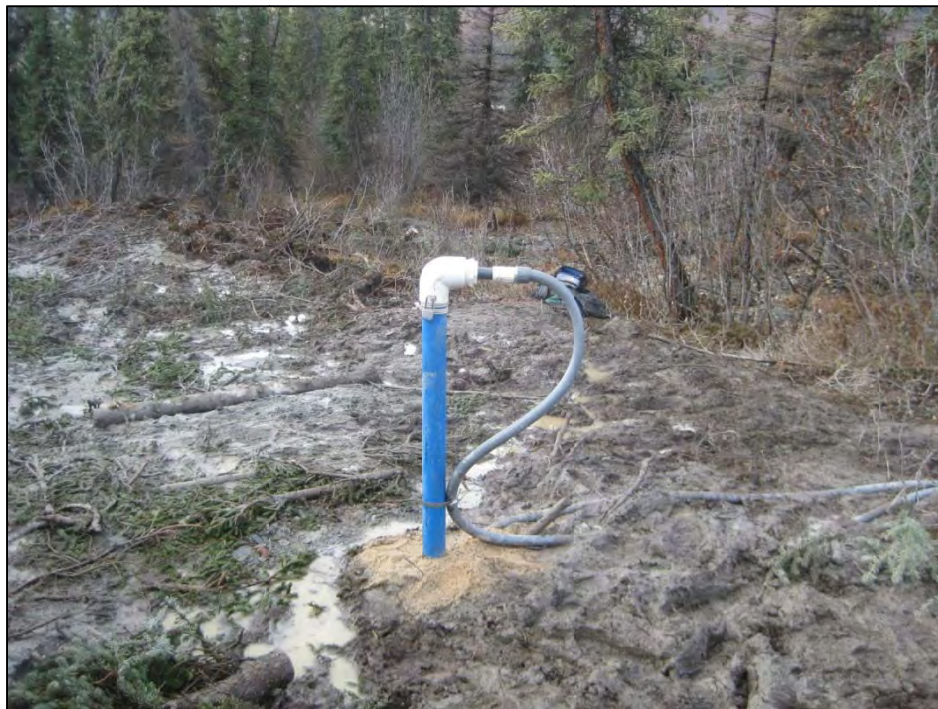
Figure D-6. Completed casing and instrument installation in TH12-9004. (Photograph by M. Darrow, Sept. 2012)
