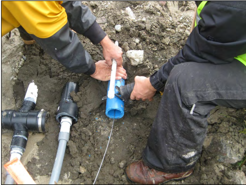
Figure C-18. Trimming the downslope guide casing for ABS end cap adapter. (Photograph by M. Darrow, July 2012)
