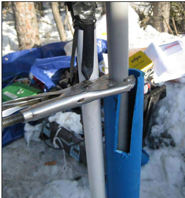
Figure A-13. Installing inner 1.05-in. PVC into guide casing for SAA device. Slot cut into the guide casing was to allow tightening of the hose clamp at the top of the PVC casing (see Figure A-14). White 1-in. PVC to the left was for a thermistor string. (Photograph by M. Darrow, March 2010)
