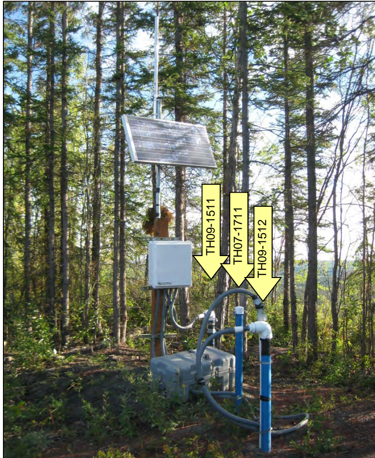
Figure 4. Relative locations of the measured casings at Rich113. Vertical arrows are labeled with the test hole identifiers. The edge of the bluff overlooking the Copper River is immediately beyond the spruce trees behind the installations, and the Richardson Highway is behind the photographer. (Photograph by M. Darrow)
