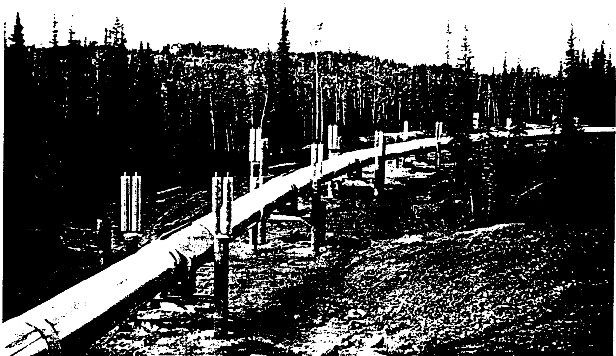
Figure 3. McDonnell Douglas "Cryoanchor" thermosyphons used on TAPS in Alaska.
