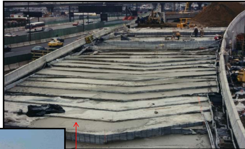
CALTRANS LA Bridge Approach
