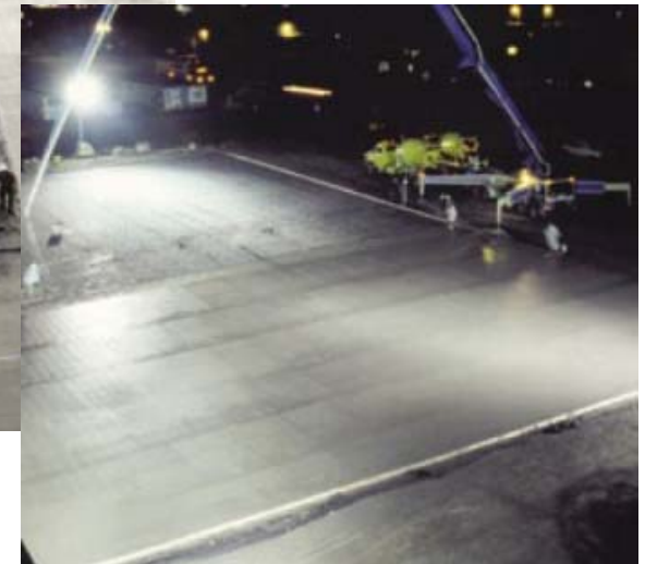
Exterior Concrete Pavement Atlanta Bonded Warehouse Corp. – Kennesaw, GA - 1993
