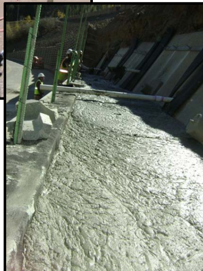
Pervious fill behind lower bin wall
