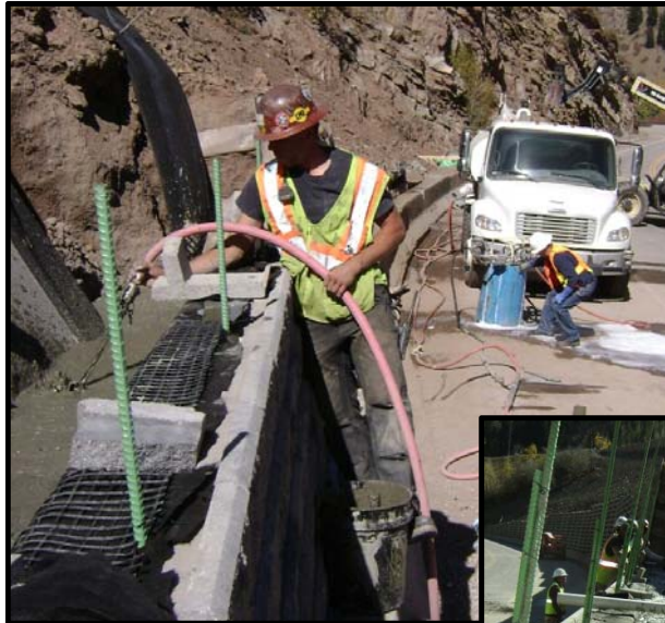
Pervious fill behind lower bin wall
