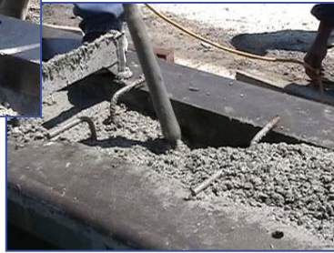
Vibrated Concrete with 6.5 in. slump
