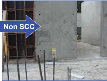
7 in. slump vibrated concrete
