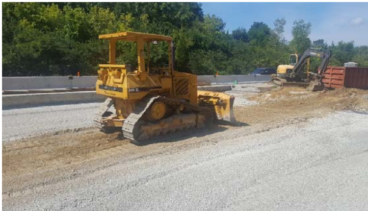
Sinkhole remediation in the median
