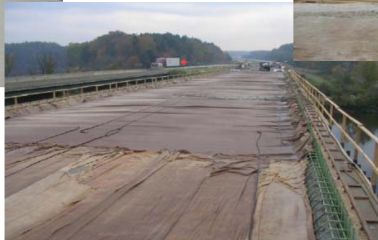
I 80 Ohio Turnpike Meander Creek, OH 2006
