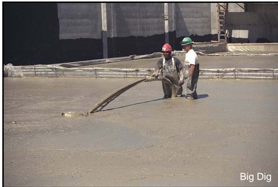
Subgrade Stabilization
