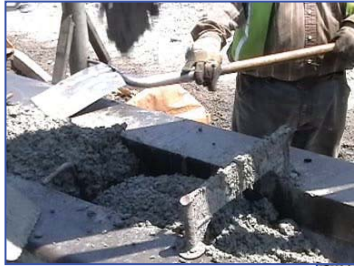
Vibrated Concrete with 6.5 in. slump
