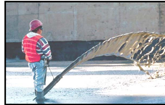
Cellular Concrete has been pumped over 700 feet vertically and over 17,000 feet
