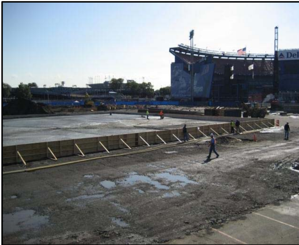
The site of the new ball park is on organic clay
