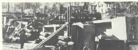
(c) Girder after failure.
