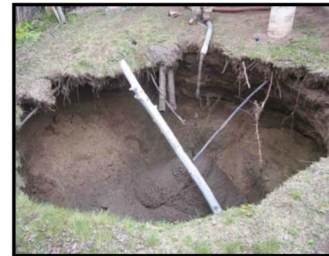
Damage from 2005 subsidence event
