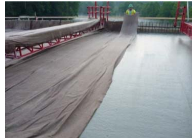
Wet curing a VA bridge deck to ensure maximum designed expansion
