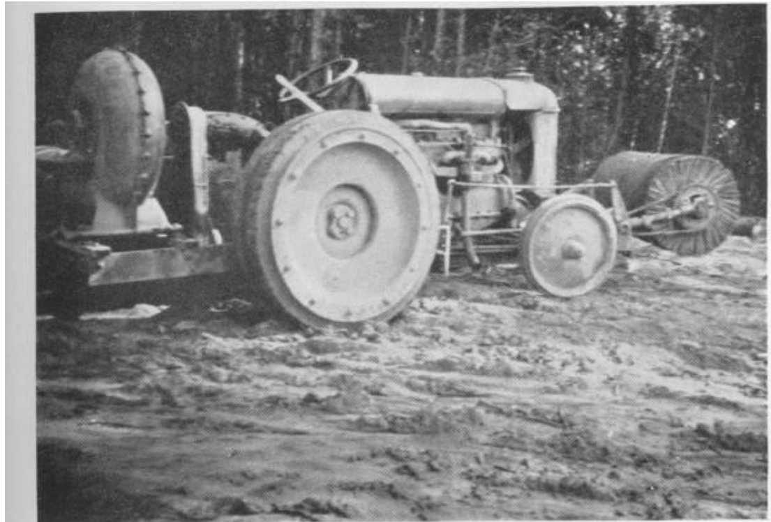
ROAD CLEANING EQUIPMENT, SHOWING BROOM AND BLOWER MOUNTED ON A FORDSON TRACTOR. THE BLOWER REMOVES THE DUST THAT HAS NOT BEEN ENTIRELY SWEEPED OFF BY THE BROOM.
