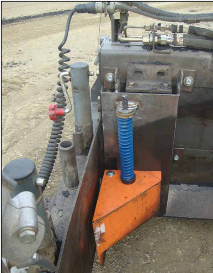
Safety Edge shoe with modified back plate
