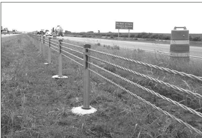
Below: A high-tension four-strand cable median barrier.
