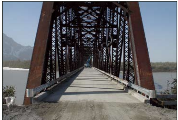
A new concrete deck was poured to replace the old deck.
