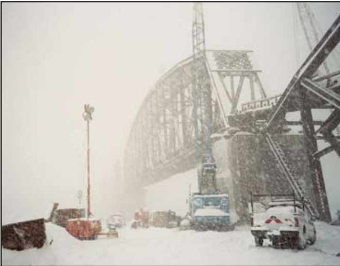
Weather conditions during the repair were not always good.
