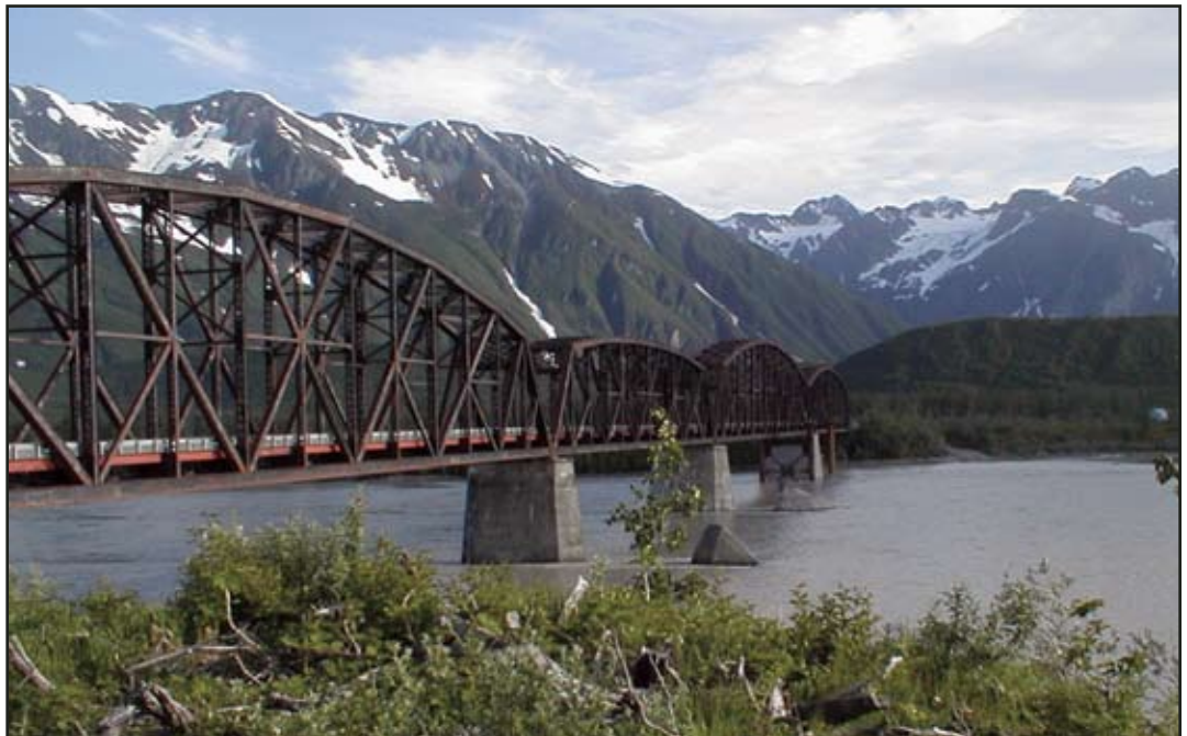
The profile of the Million Dollar bridge is restored 41 years after the 1964 earthquake dropped the north span off its pier (below).
