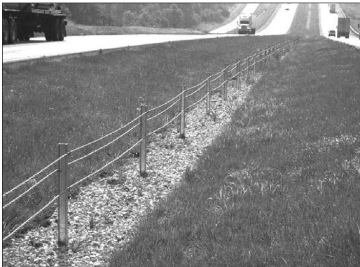
Above: A standard three-strand cable median barrier.
