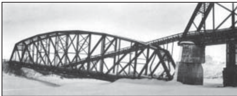
The Miles Glacier Bridge, now called The Million Dollar Bridge, was built by the Copper River and Northwestern Railway and finished in 1910. The Territory of Alaska took possession of it in 1945. The photo shows its present condition after the northernmost of four spans, was knocked off the pier in the 1964 earthquake. The auto ramp was added in 1973.
