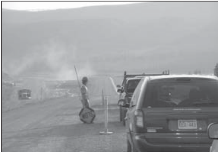
This flagger may be confusing the motorists by letting the sign drop. No positive direction is given to either stop, or proceed slowly.
