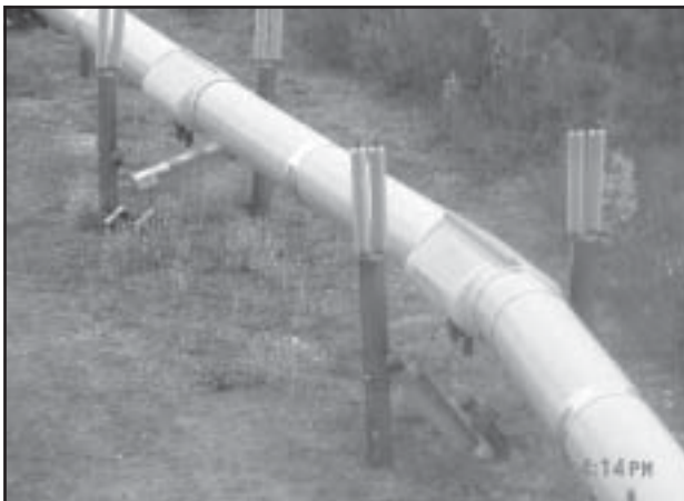
Damage to the Trans-Alaska Pipeline included collapsed crossbars on the vertical support members
