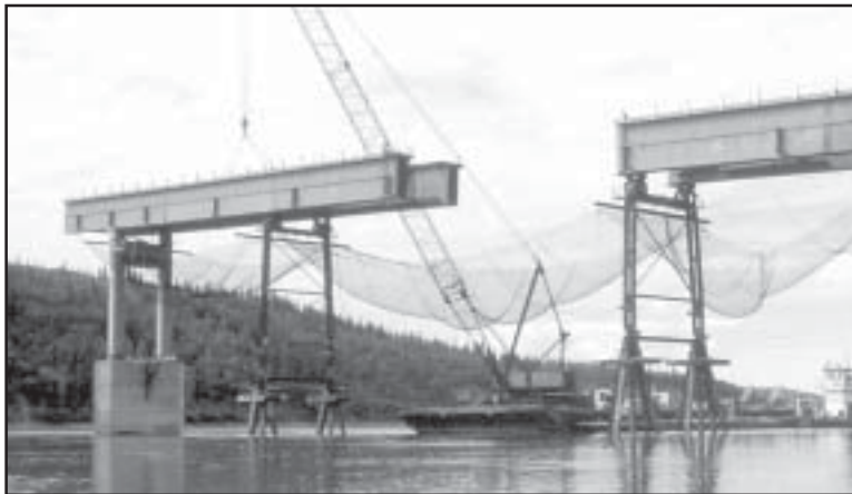
A barge lifts a steel bridge girder into place in June 1975, during construction of the Dalton Highway. This highway was built to access the northern part of Alaska for construction and then maintenance of the Trans-Alaska Pipeline Project, which was completed in 1977.
