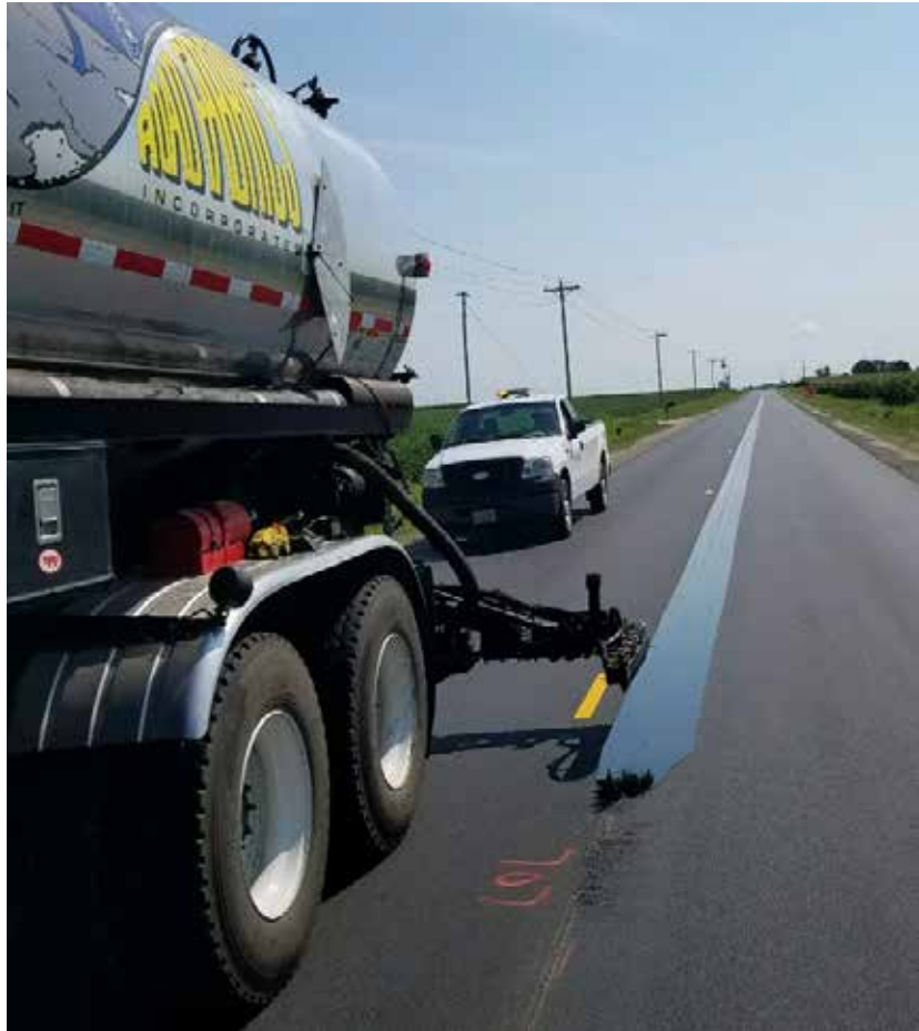
Placed by pressure distributor with mechanical agitation in tank
