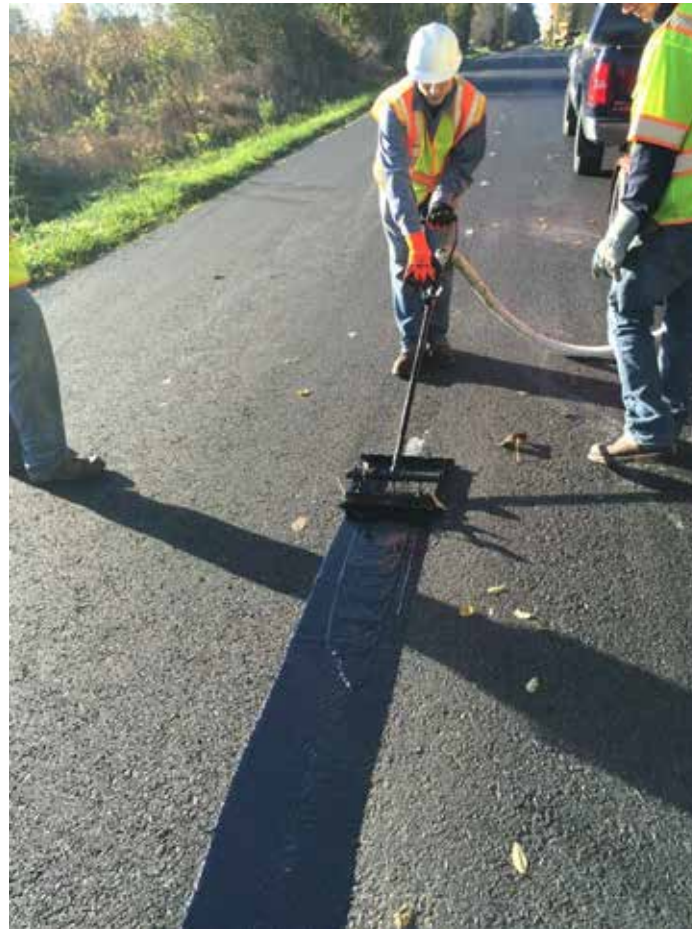
Manual strike off box fed from melting kettle
