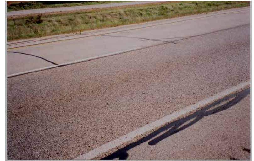
Conventional Asphalt Mix vs. SMA
