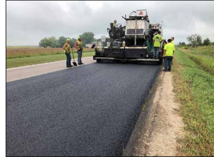
Newly Paved Ultra-Thin Bonded Wearing Coarse (UTBWC) Section Source: MnDOT 2022
