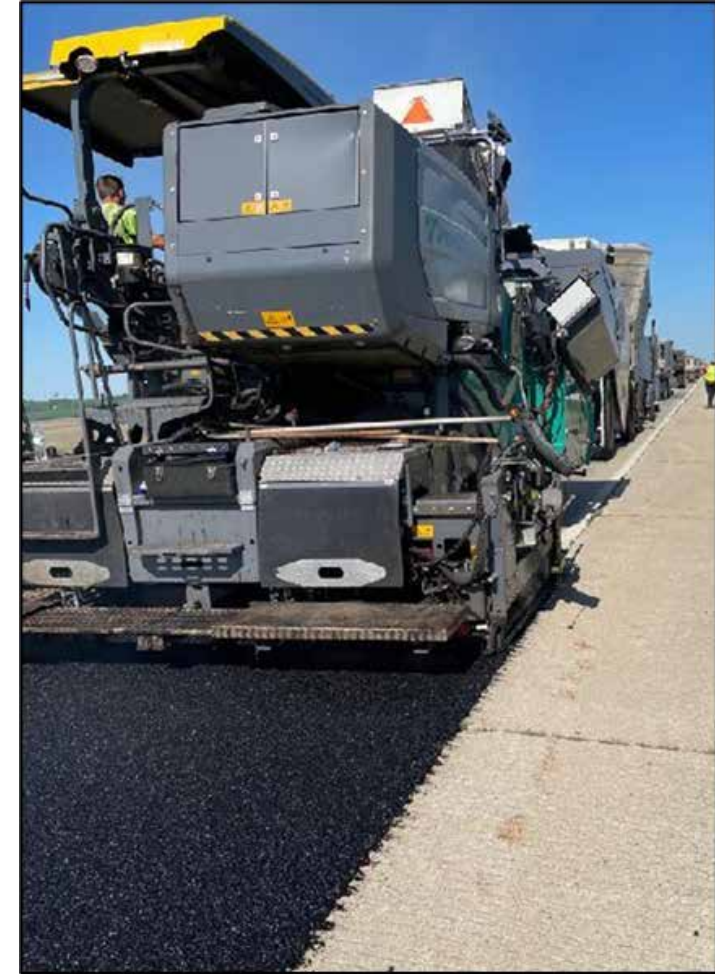
Source: Asphalt Surface Technologies Corporation
