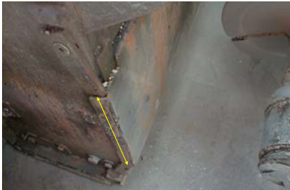
Moves up and down tamping mix under the screed
