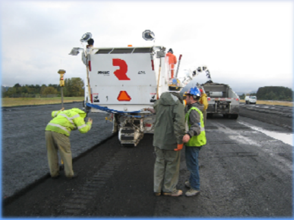
Milling to Finished Grade
