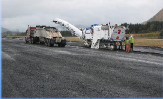
Milling to Finished Grade
