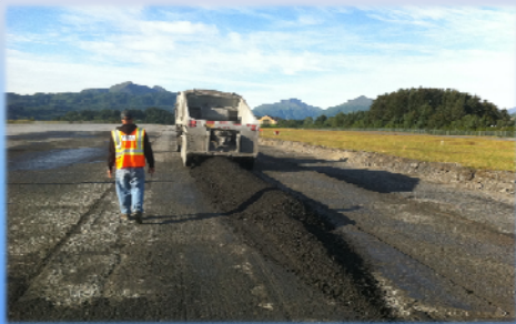
Placing the Foamed RAP
