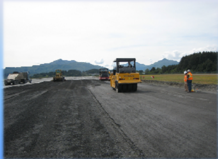
Compaction with Smooth Drum and Pneumatic
