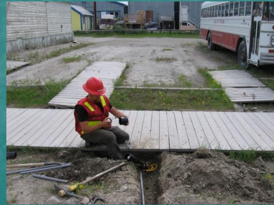
Installing Thermistor
