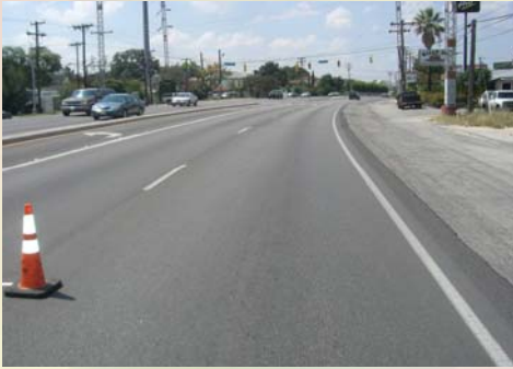
No Distress Evident after One Year of Service
