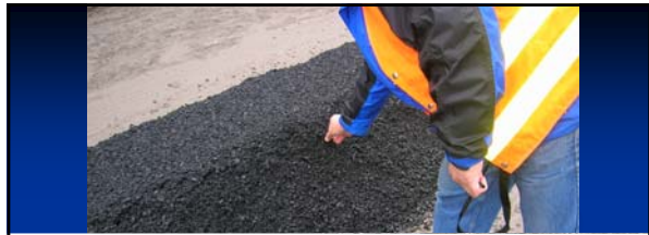
Beginning of Construction
