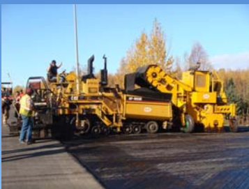
Cat AP-1055B paver & Weiler E650 pickup machine
