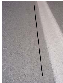
1996 - Pittman Rd. Turn Lane
