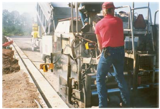
Track a Curb
