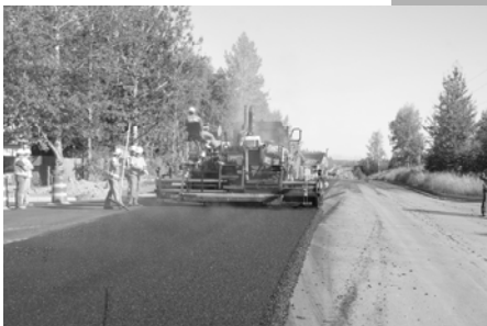
South end of project: 3-inch lift
