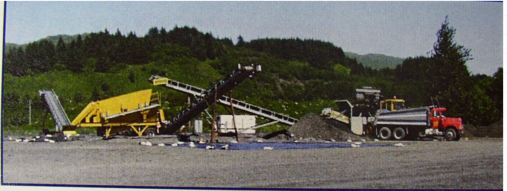
Thunderbird screening plant used to screen oversize materials from contaminated soils.
