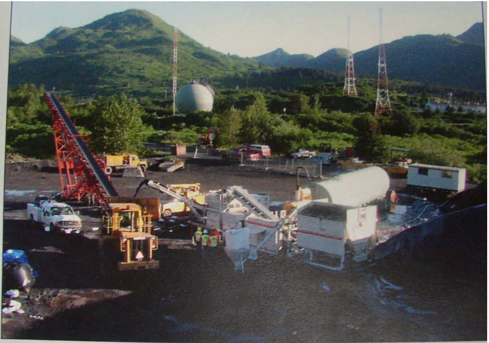
Producing foamed ATB using stationary mixing plant, July 2003.
