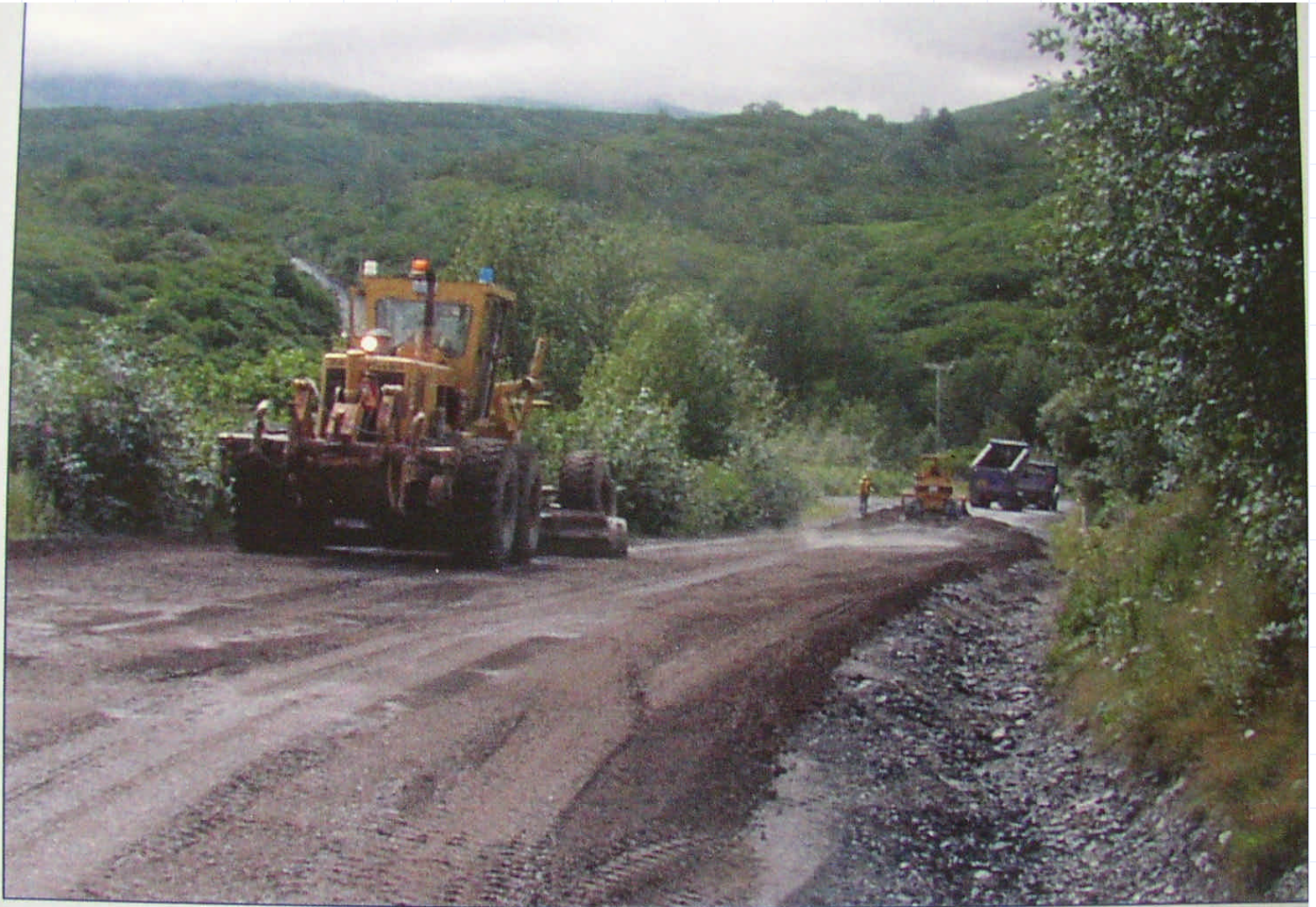
Placing foamed ATB near Mile 15 of the Rezanof Highway, July 2003.
