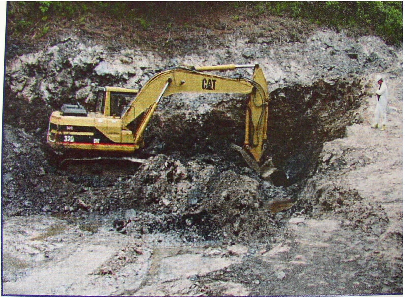
Excavating contaminated material at the ADA site.
