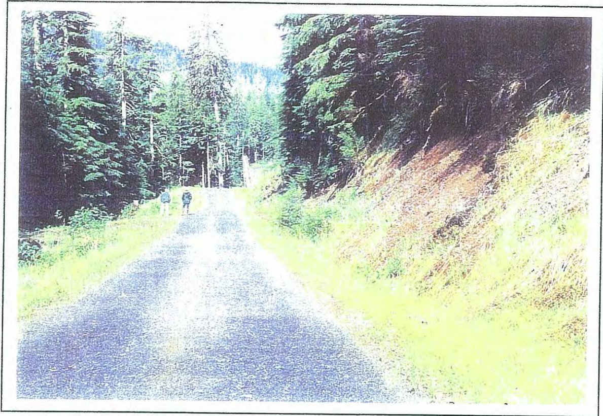
Photo 3 : Close-up of typical steep cut construction in common material. Note steep brow at top of cut.
