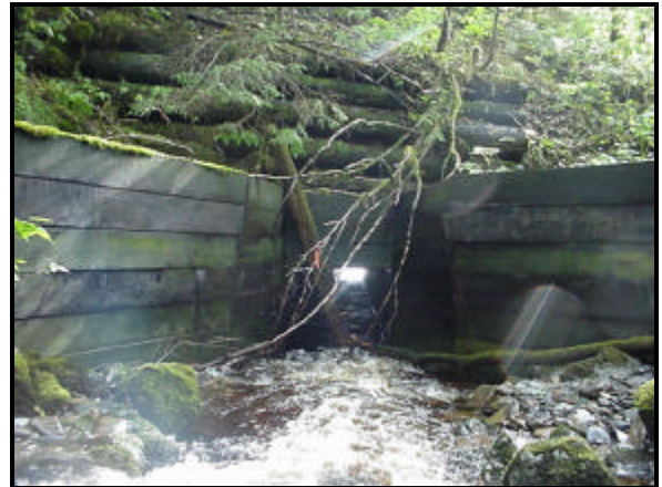
Figure 17 - Auke Nu Creek entering culvert under Glacier Highway
