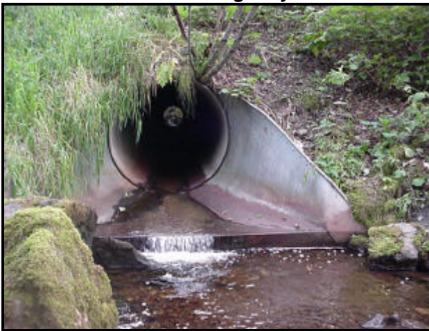
Figure 10 - Bay Creek exiting culvert under Glacier Highway
