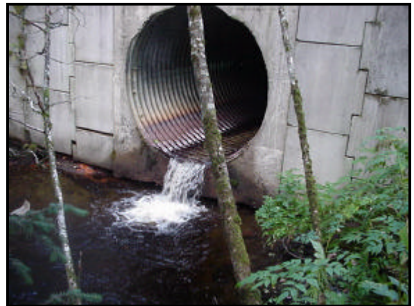
Figure 15 – Waydelich Creek exiting culvert under Glacier Highway
