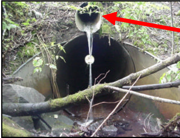
Figure 8 - Bay Creek entering culvert under Glacier Highway
