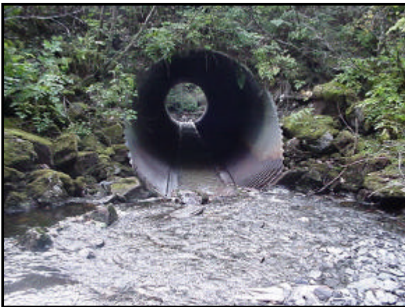
Figure 14 – Waydelich Creek entering culvert under Glacier Highway
