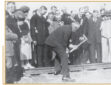
President Harding driving in golden spike that completed the Alaska Railroad; Nenana, July 15, 1923
