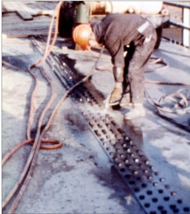
Figure 6-4. Splice Plates and Bolts below Timber Wearing Surface
