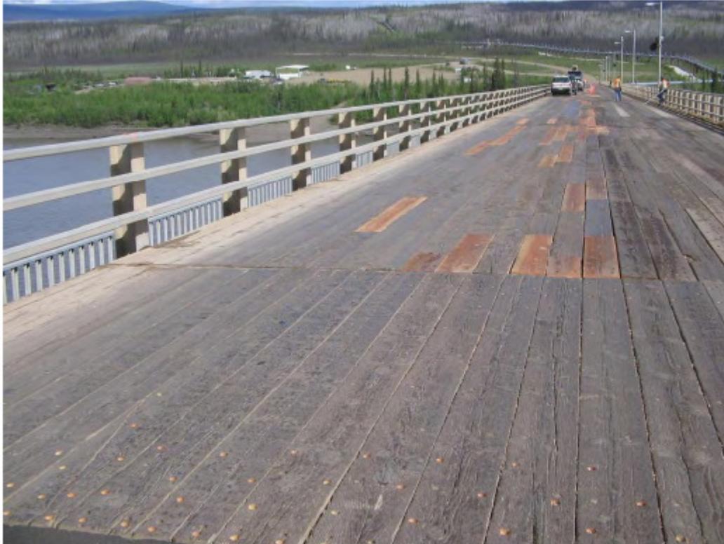
Figure 1.1 Timber deck repair, a maintenance activity.
