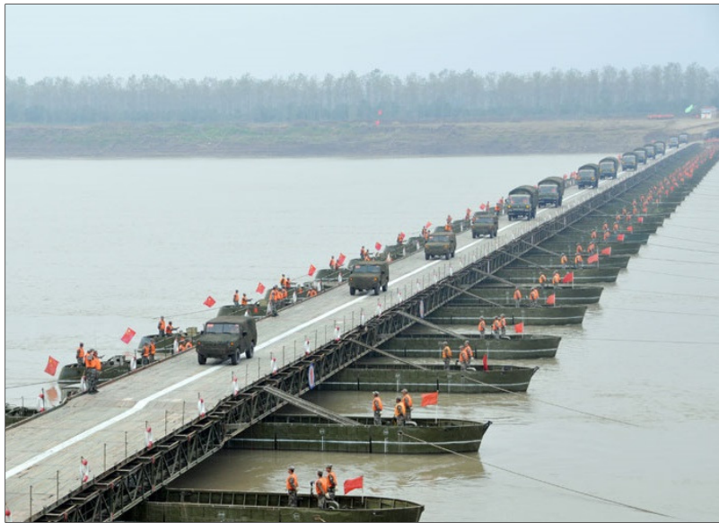
Figure 6-11. Temporary Floating Bridge Example
