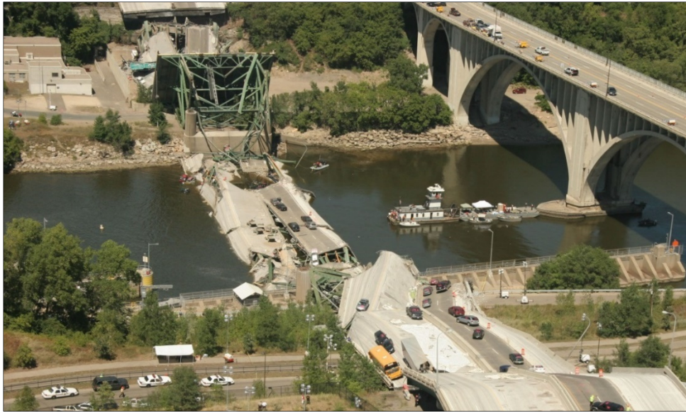
Figure 6-1. Fracture Critical Bridge Failure in Minneapolis
