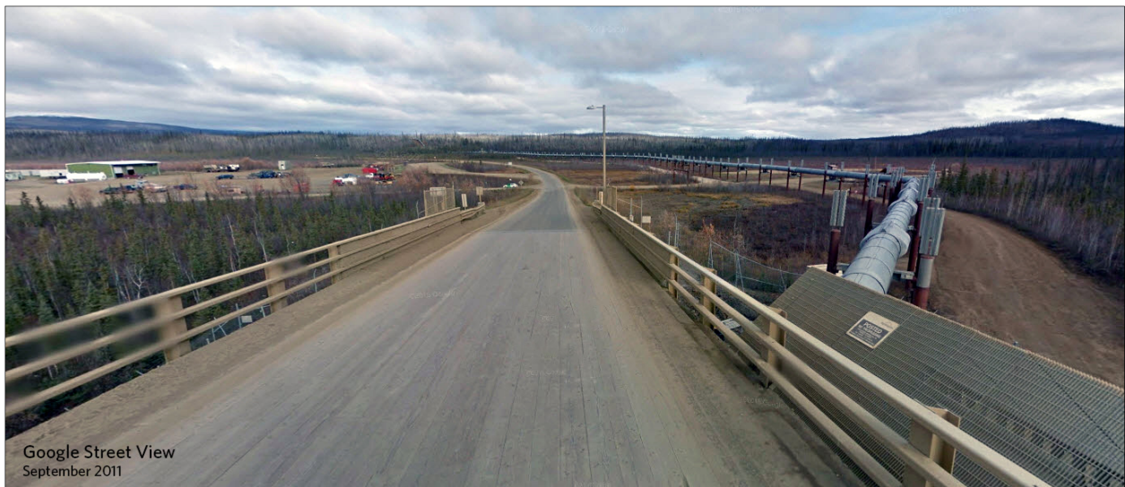
Figure 2-4. Yukon River Bridge Crossing, Looking Northbound, 2011
