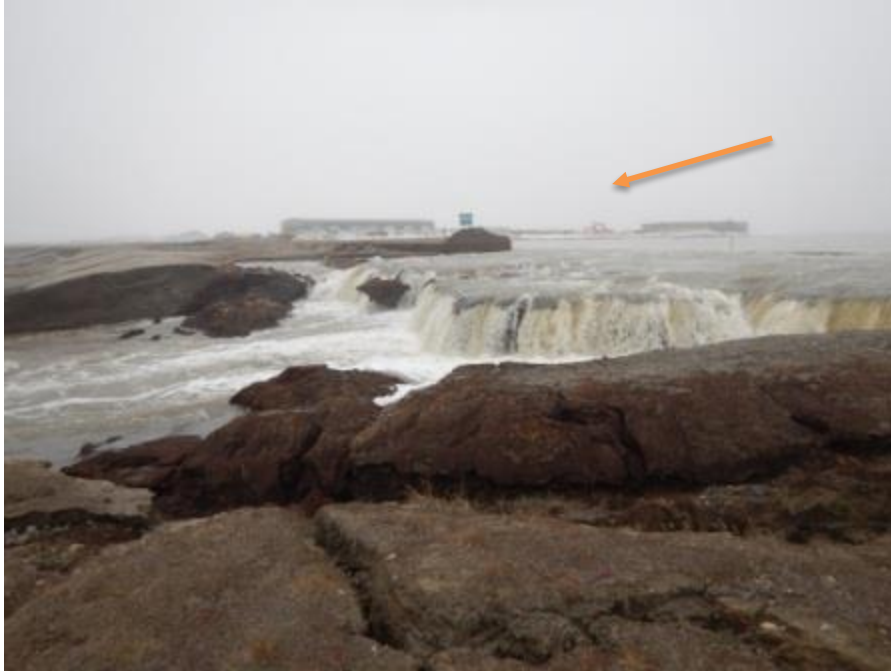
Figure B.3. Photo taken May 22, 2015, near Dalton Highway MP414, view south. This photo was taken several feet to the right of Figure B.2. Note the extensive removal of permafrost in center of photo and continued erosion at the waterfall face. The difference in elevation from tundra surface to the active river channel is approximately 9–12 ft (3–4 m) in this area.
