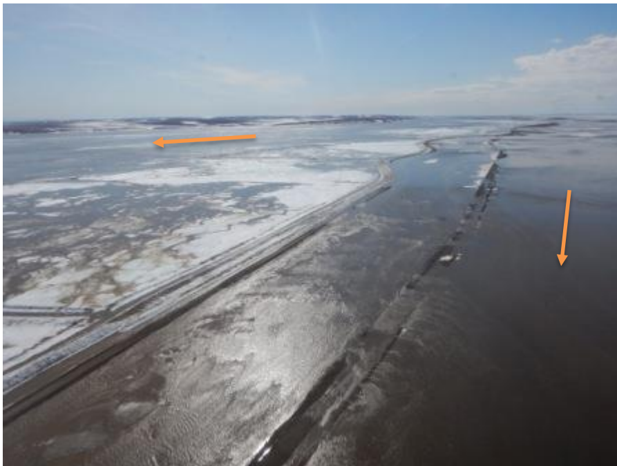
Figure B.6. Photo taken May 19, 2015, near Dalton Highway MP400, view south. Continued high water west (right) of the road and pipeline. A Sagavanirktok River channel is at far left, and Franklin Bluffs appear near the horizon, upper center of photo.
