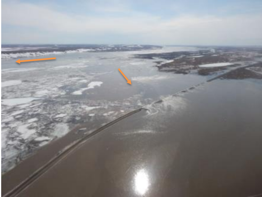
Figure B.21. Photo taken May 21, 2015, near Dalton Highway MP395, view southeast. Much aufeis at left is exposed, and water levels are falling. Eroded channels across road are clearly visible. Franklin Bluffs seen in upper left.
