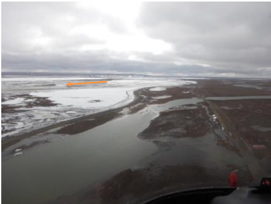
Figure B.10. Photo taken May 31, 2015, near Dalton Highway MP400, view south. Tundra between road and pipeline is emerging as water levels continue to fall. The aufeis between the road and pipeline is completely gone, but much remains east (left) of the road. Road repair work has begun. A Sagavanirktok River channel is at far left, and Franklin Bluffs are seen on the horizon, upper left of center.
