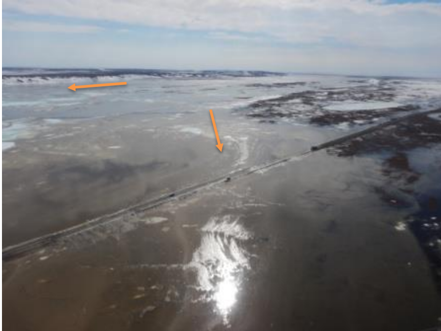
Figure B.17. Photo taken May 17, 2015, near Dalton Highway MP395. View is southeast and shows the initial flooding of the road in this area. This location is the southernmost incidence of flooding during this event. Compare with Figure B.14, which shows a ground view as seen from the road surface at left edge of this photo. Note vehicles still using road. Franklin Bluffs are in the distance.
